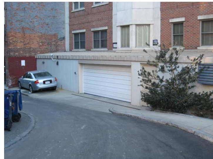
View of the rear elevation concrete walkway and parking garage entrance apron adjacent to Public Alley #904.
