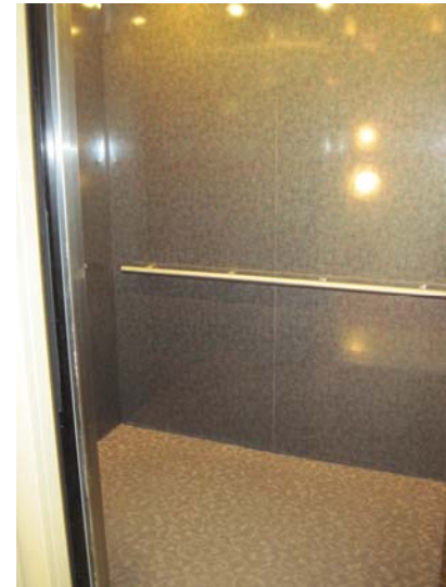
View of the elevator finishes. High-gloss laminated particleboard panels with stainless steel trim and carpeted floors.
