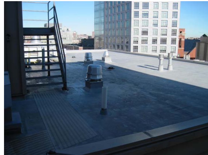
All roof surfaces feature mechanically fastened thermoplastic polyolefin (TPO) roofing systems.
