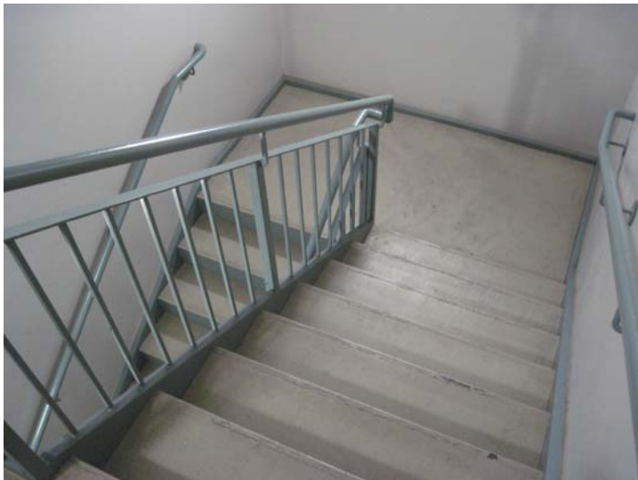
Both stairwells feature poured concrete treads with metal stringers, risers, and railings, and (???)
