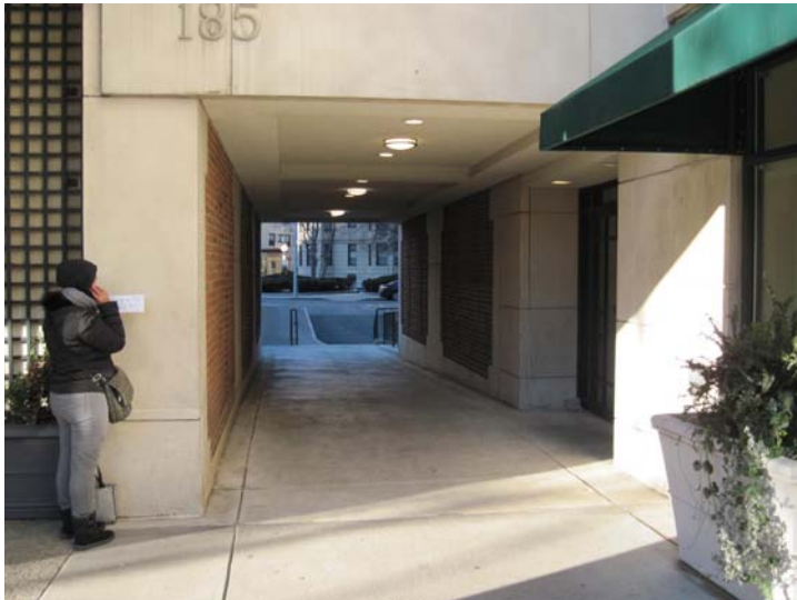
Limited site elements include this concrete walkway leading from the front Massachusetts Ave elevation to the rear elevation and public alley.
