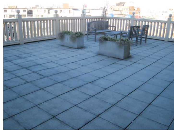
View of the 9 th Floor rooftop common-use terrace with pre-cast concrete tile decking.
