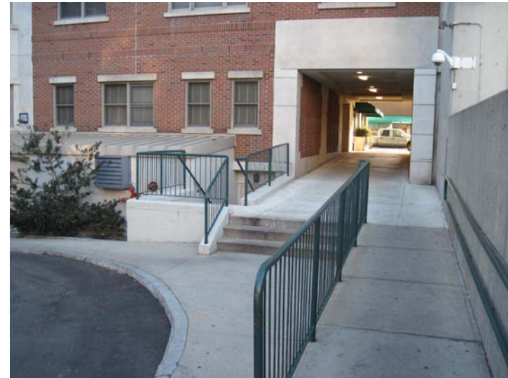
View of the rear elevation concrete walkway, steps, ramp, and painted metal railing.
