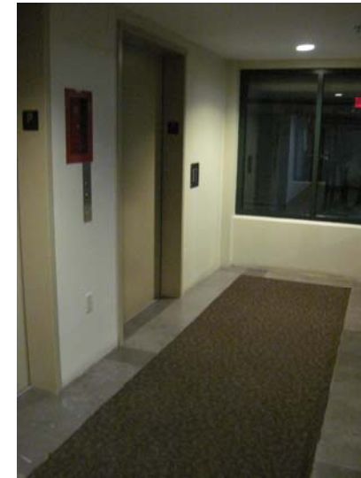
View of the garage elevator lobby finishes. Painted wall and ceiling surfaces, granite tile floor.
