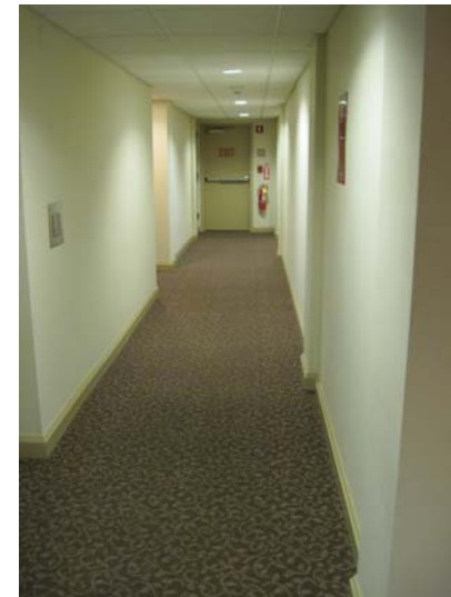
View of typical hallway finishes at floors 2 through 8; painted drywall walls, acoustic tile ceiling, and carpeted floors.
