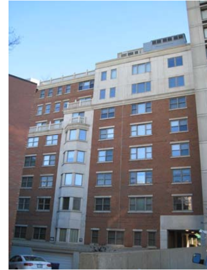
View of the rear (west) elevation.
